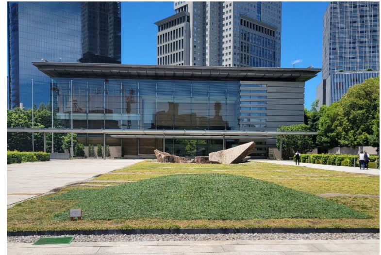
View of the post-construction
