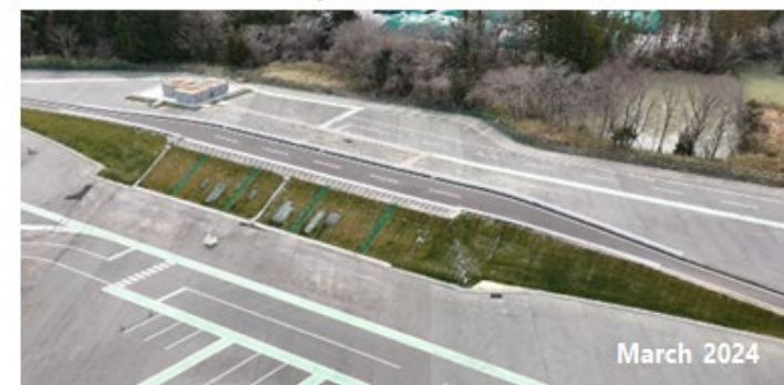
Road embankment demonstration project in the premise of the ISF
