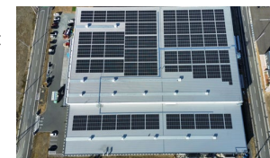
Support for the introduction of photovoltaic power generation facilities on a factory rooftop (Minamisoma City) (FY2024 Project)
