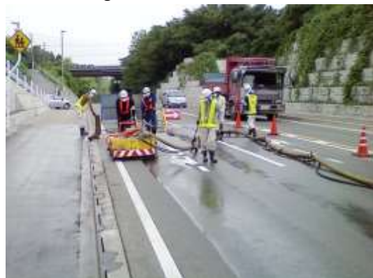
Credit: Maeda Corporation Extra high-pressure washing
