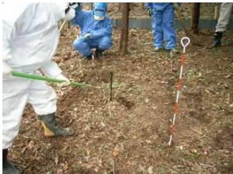
Removal of organic residue by metal rake
