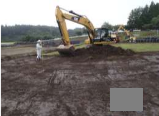
Credit: Shimizu Corporation Topsoil scraping
