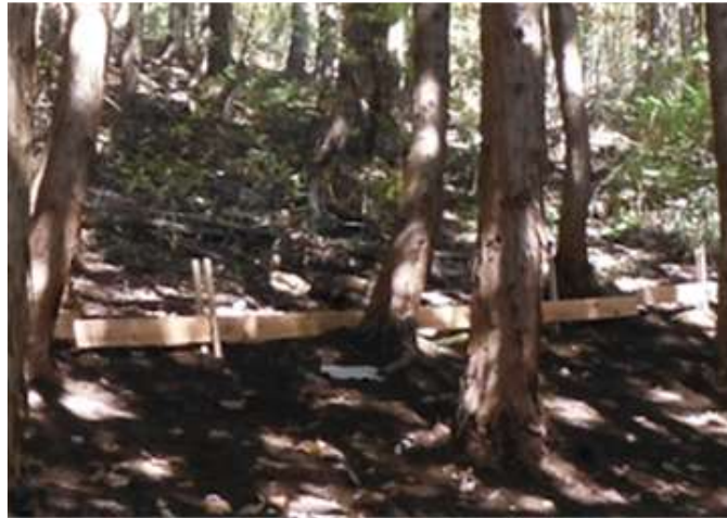
Fig. 4-22 Example of measures including decontamination of forests (measures to prevent soil runoff)
