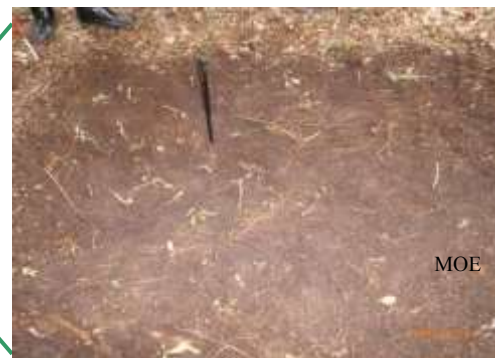
Ground surface after removal of organic residue (roots start to be exposed).
