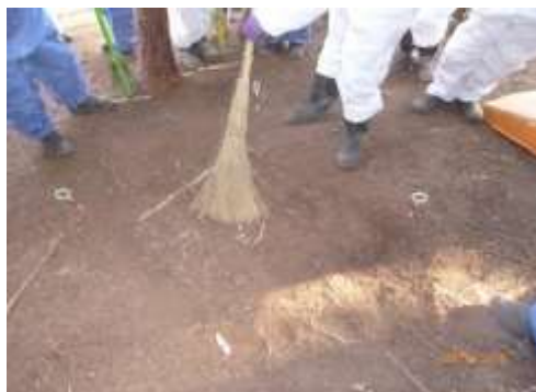
Removal of residue by bamboo broom* after removal of organic residue * Cut to about 20 to cm to ensure flexibility of tip.
