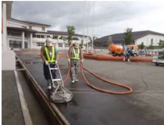
Credit: Taisei Corporation High-pressure water washing
