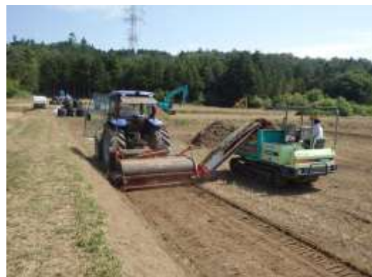
Credit: Hazama Ando Corporation Topsoil scraping and collecting using specialized equipment
