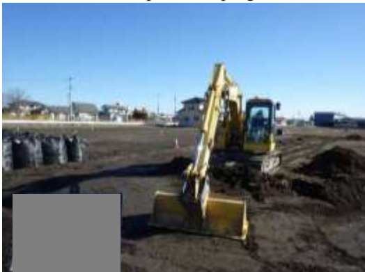
Credit: Hazama Ando Corporation Topsoil scraping and collecting using specialized equipment
