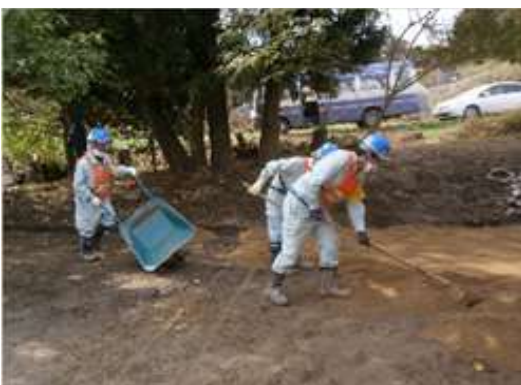
Credit: Taisei Corporation Covering with topsoil
