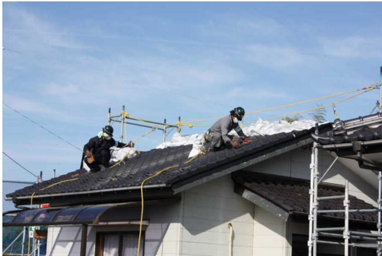
Decontaminating roofing tiles (by wiping)
