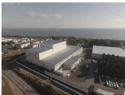
Temporary incineration facility at Okuma
