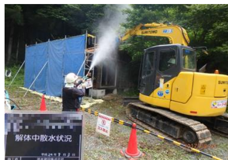
Dismantling of a damaged house
