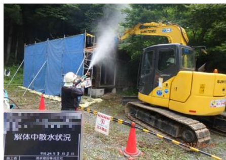
Dismantling of a damaged house
