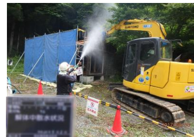
Dismantling of a collapsed house
