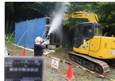
Dismantling of a collapsed house
