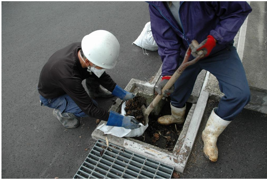
Figure 2-23. Example of the decontamination of a street drain (removal of sediments)
