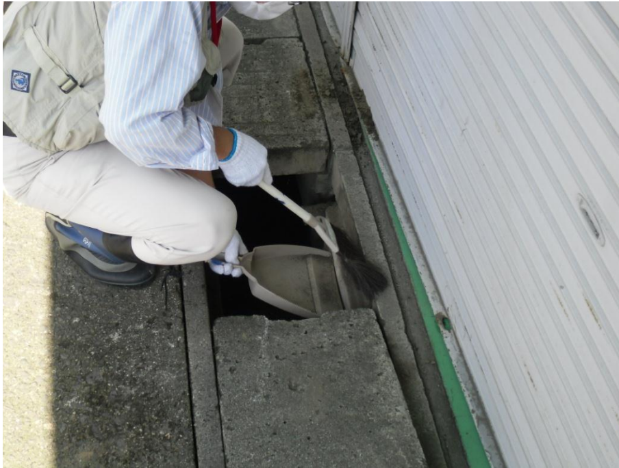
Figure 2-41: Example of decontamination of street drains (sweeping up dirt and dust)
