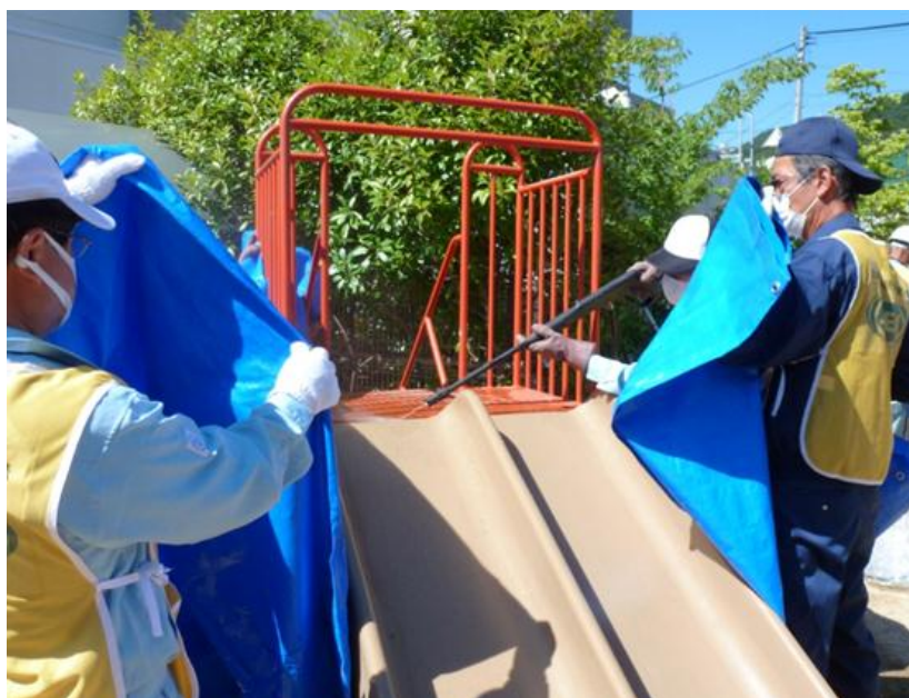
Figure 2-17. Example of decontamination of playground equipment (high pressure water cleaning)
