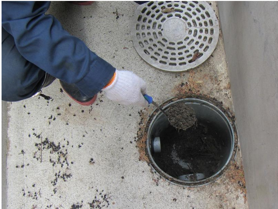
Figure 2-24. Example of the decontamination of a rainwater chamber (removal of sediments)
