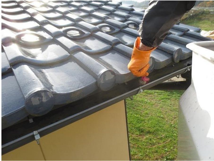
Figure 2-13. Example of the decontamination of rainwater guttering (brush cleaning)
