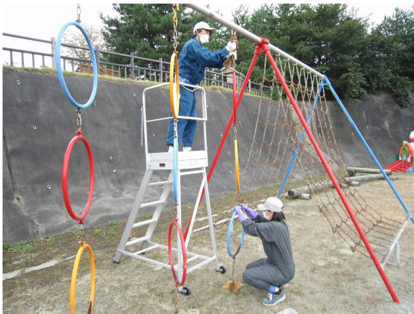
Figure 2-16. Example of decontamination of playground equipment (wiping)
