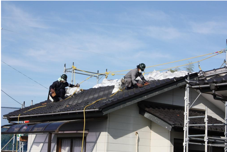
Figure 2-9. Example of the decontamination of roof tiles (wiping)
