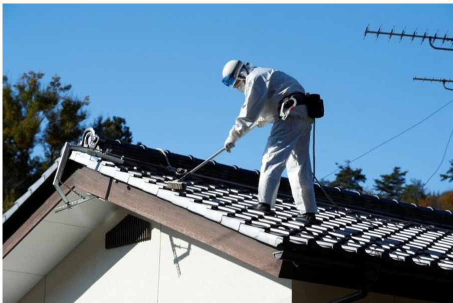
Figure 2-10. Example of the decontamination of roof tiles (cleaning)
