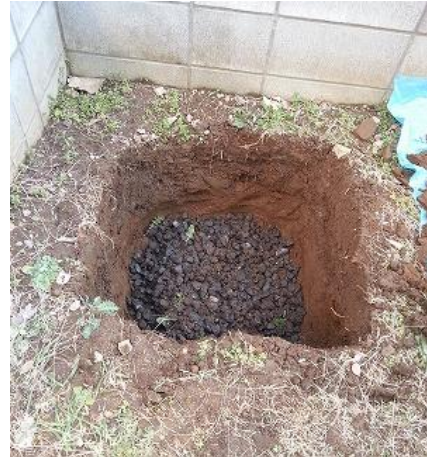
Figure 2-25. Example of the decontamination of a rainwater chamber (removal of sediments and deep plowing of the rainwater chamber sediments at the same site)
