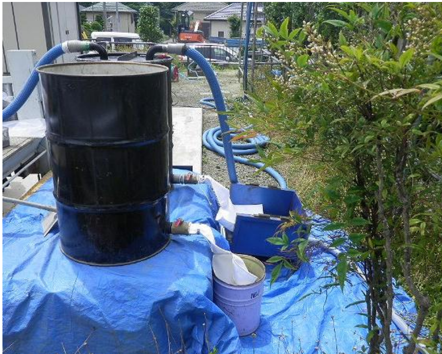
Figure 2-32. Example of wastewater treatment (sedimentation treatment using water tanks)
