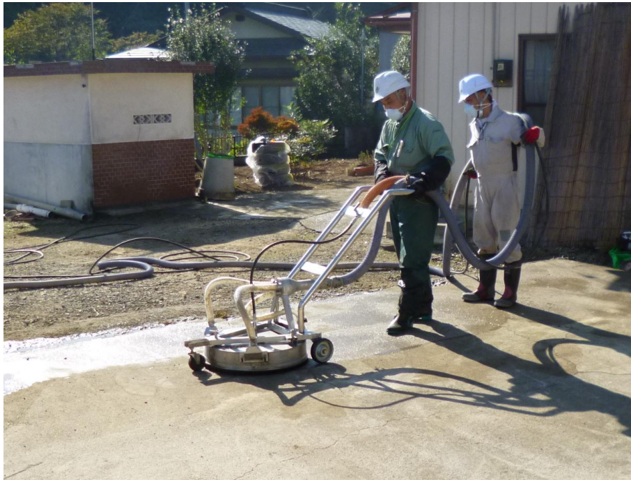
Figure 2-37. Example of decontamination of paved surfaces (water recovery-type high pressure water cleaning)
