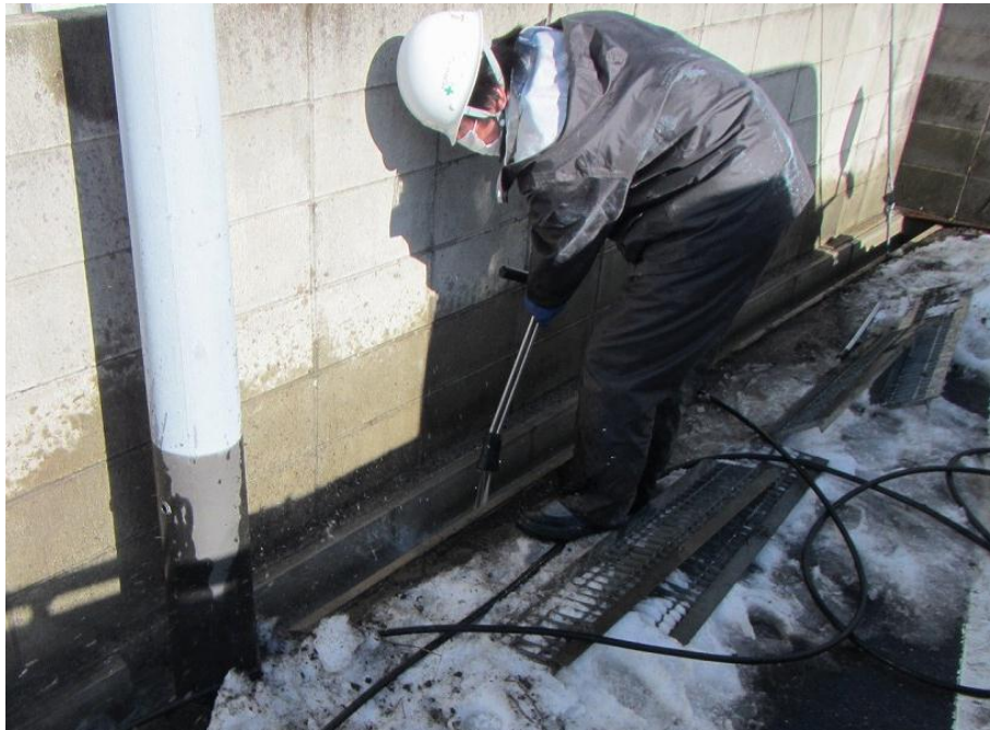
Figure 2-26. Example of the decontamination of a street drain (high pressure water cleaning)
