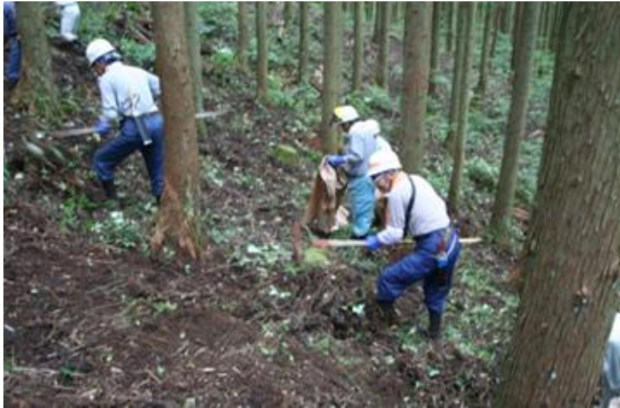
Figure 2-63: Example of the decontamination of a forest (removal of fallen leaves)
