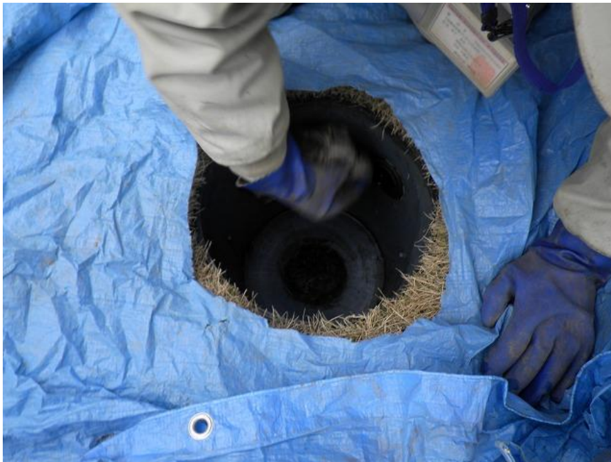
Figure 2-27. Example of the decontamination of a rainwater chamber (sponge cleaning)
