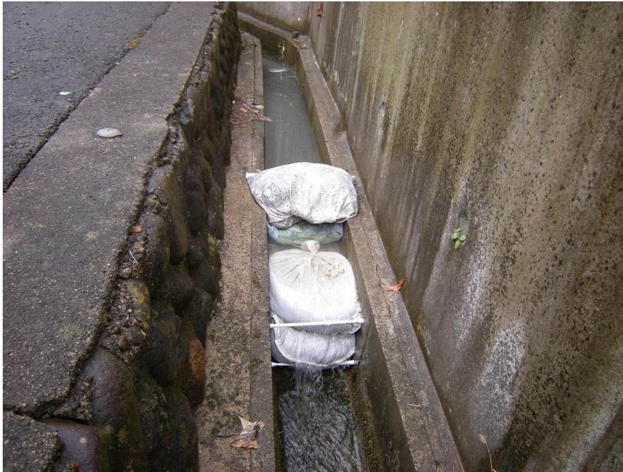
Figure 2-31. Example of wastewater treatment (sandbags installed in street drains)
