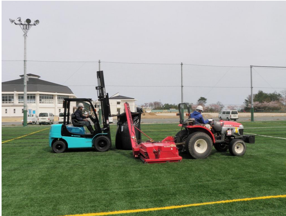
Figure 2-51. Example of the removal of infill material from artificial turf
