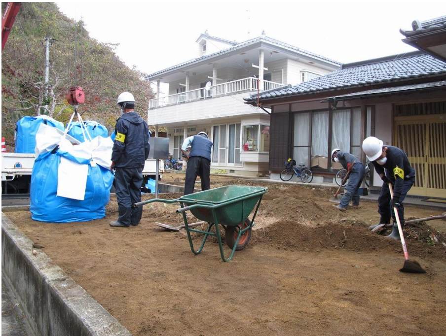
Figure 2-21. Example of the decontamination of gardens and other areas (removal of soil, etc.)
