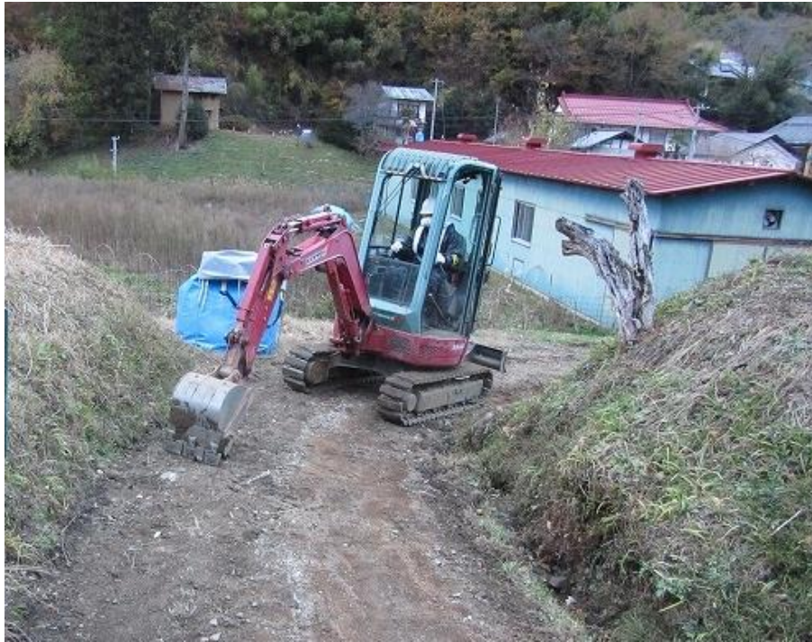
Figure 2-39: Example of the decontamination of an unpaved road (scrapping away)
