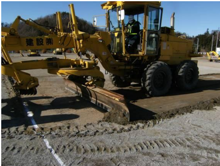
Figure 2-50. Example of the decontamination of a schoolyard (scraping away of topsoil)
