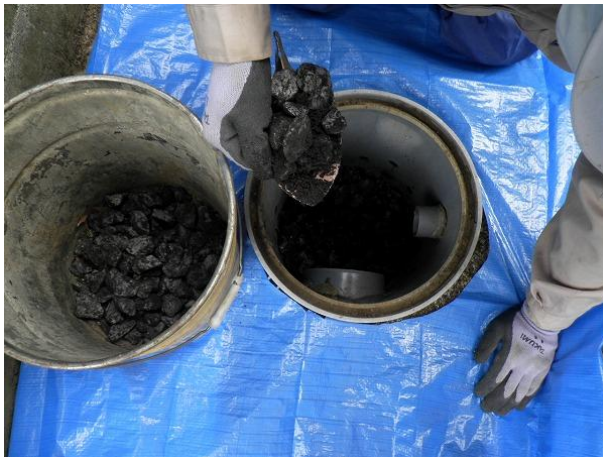
Figure 2-25. Example of the decontamination of a rainwater chamber (removal of sediments and deep plowing of the rainwater chamber sediments at the same site)
