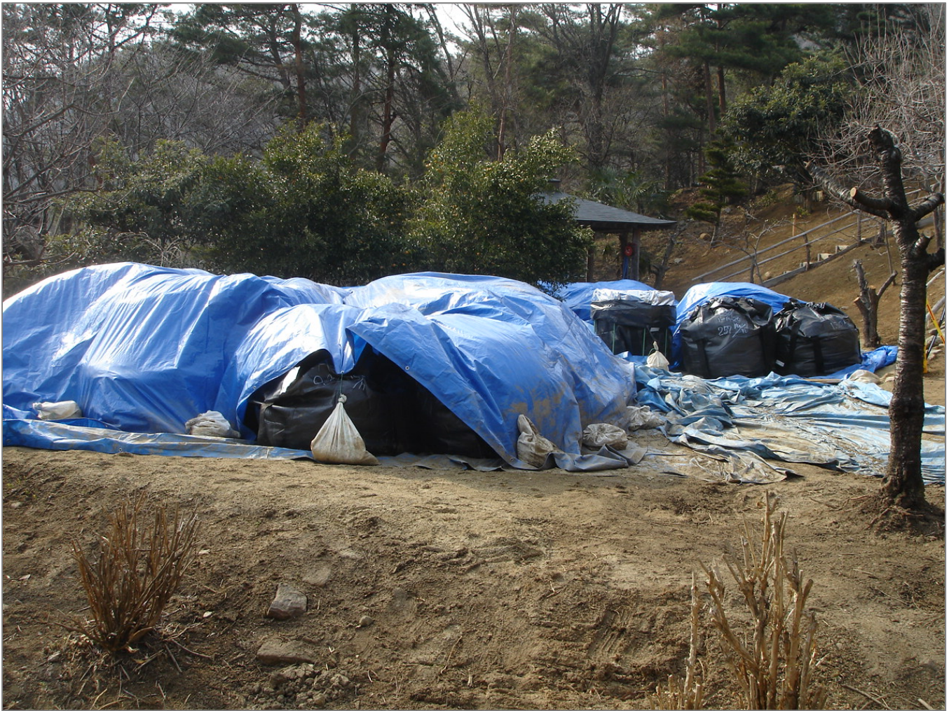
Figure 1-5 In-Place Storage at a Private Residence in Fukushima City. This storage precedes the Temporary Storage that is planned for 3-year duration to be followed by Interim Storage that is planned for 30-year duration
