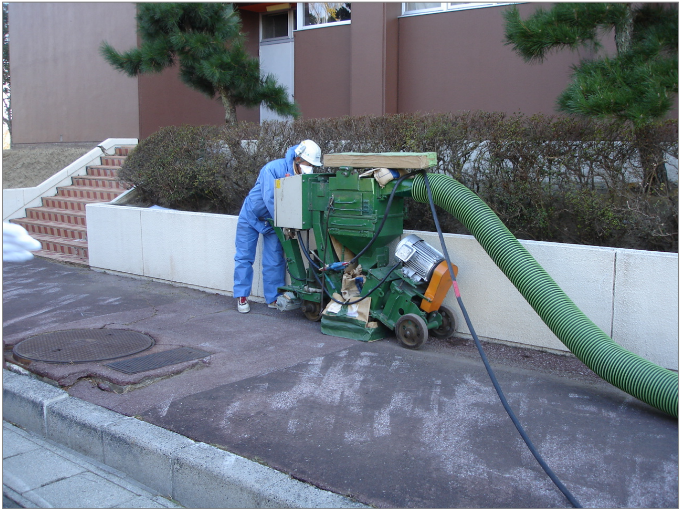
Figure 1-6 Shot-bead Cleaning of Sidewalk at the Sports Complex in Tomioka Town. This method is effective at removing near-surface with attached cesium contamination. This mature method is used in full-scale decontamination work.
