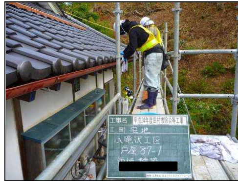
Wiping off a gutter
