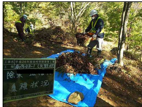
Mowing and removal of sludge
