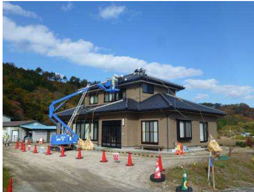
Wiping off rooftop and walls
