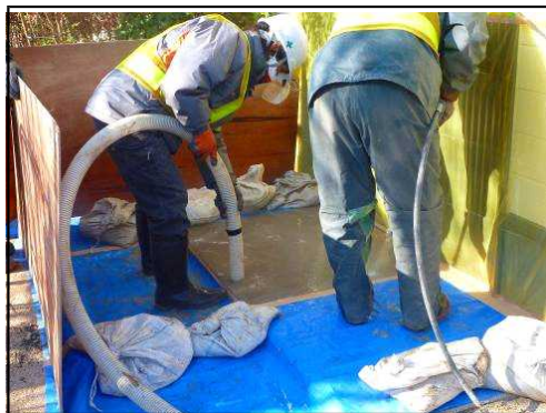
High pressure water cleaning of paved road
