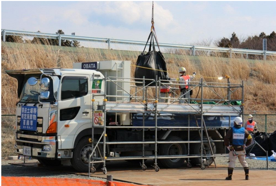
Transportation operations from Minami-Daira TSS in Okuma town
