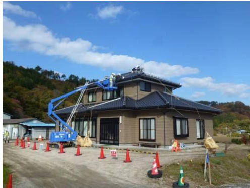
Wiping off rooftop and walls
