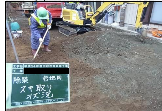
Removal of crushed stones and topsoil, and covering with clean soil
