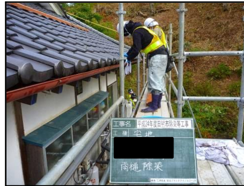
Wiping off a gutter
