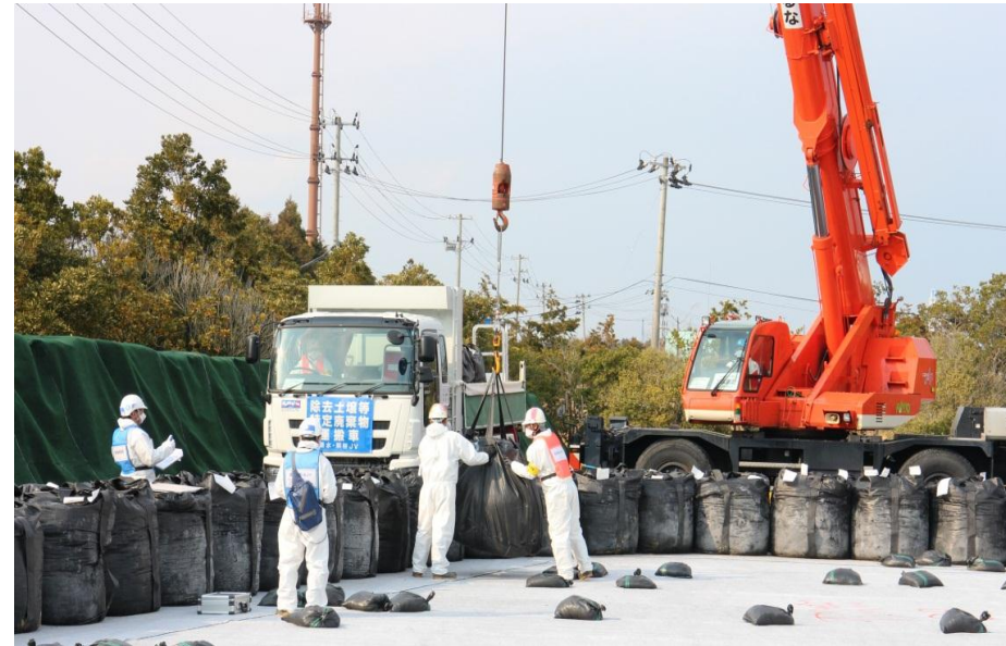
Installation operations to the stock yard in Okuma town
