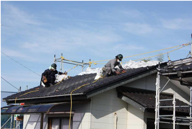
Decontaminating roofing tiles (by wiping-off)
