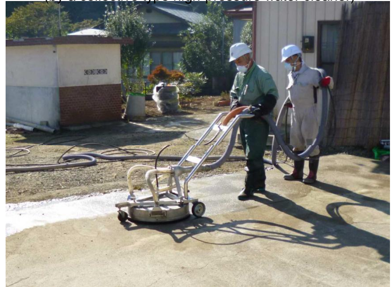
Decontaminating paved surfaces (by a collective type high-pressure water cleaner)
