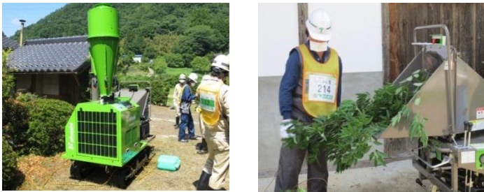
Chipping operation in decontamination site
