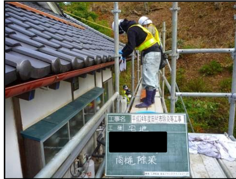
Wiping off a gutter
