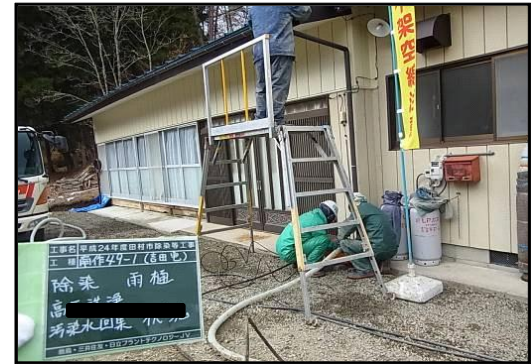
High pressure water cleaning of a drain pipe
