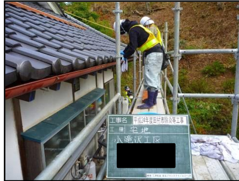
Wiping off a gutter
