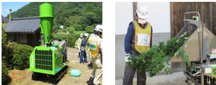
Chipping operation in decontamination site
