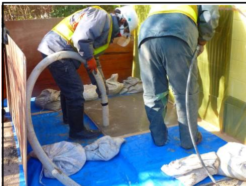
High pressure water cleaning of paved road
