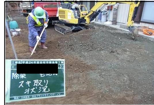
Removal of crushed stones and topsoil, and cover with clean soil
