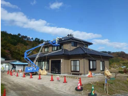
Wiping off rooftop and walls
