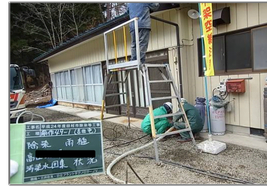
High pressure water cleaning of a drain pipe
