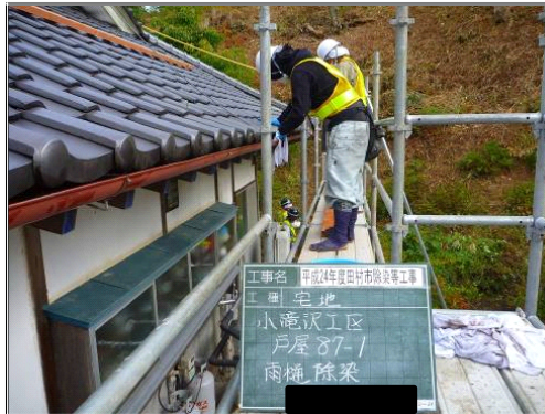
Wiping off a gutter
