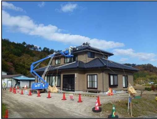
Wiping off rooftop and walls
