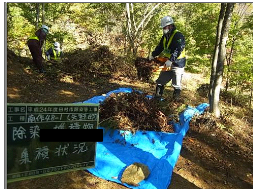
Mowing and removal of sludge
