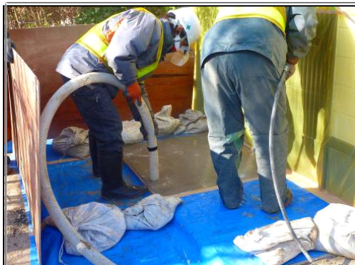
High pressure water cleaning of paved road
