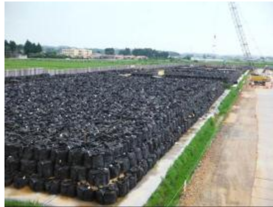
Installing in Nagano temporary storage site in Minami-Soma
