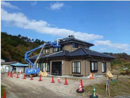
Wiping off rooftop and walls
