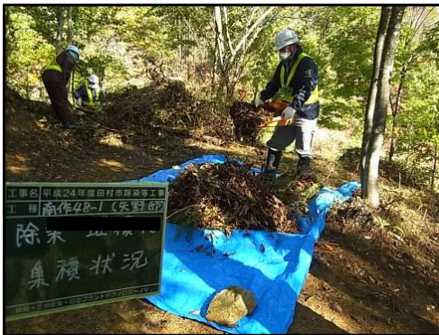
Mowing and removal of sludge
