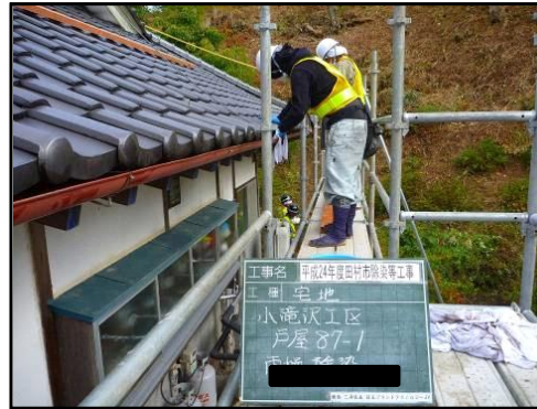
Wiping off a gutter
