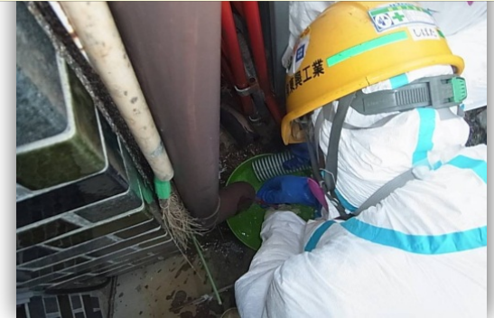
Gutter (vertical): high-pressure water cleaning
