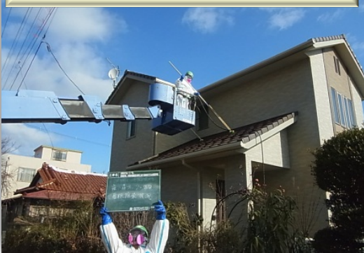
roof: water cleaning, cleaning with brush
