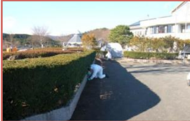
Thorough removal of soil on asphalt surface
