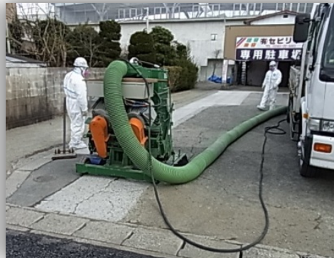
Concrete floor: Shot blast
