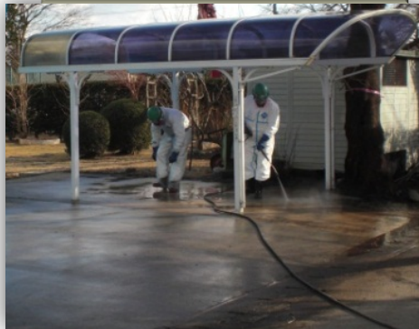
Concrete floor: High-pressure water cleaning
