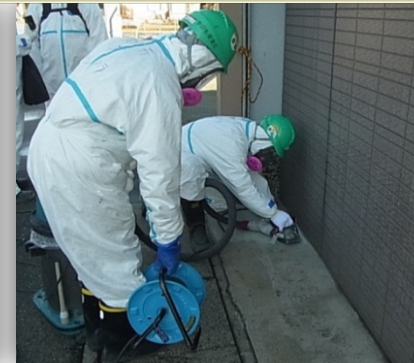
Concrete floor: Surface grinding machine
