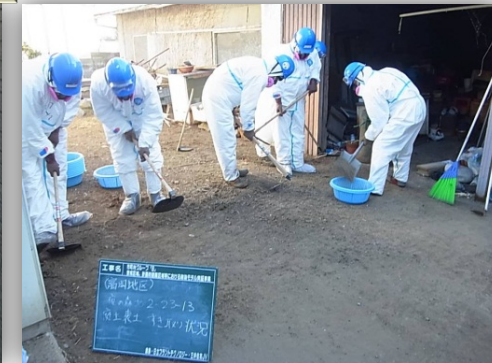
Garden: removal of topsoil
