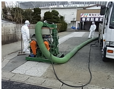
Concrete Slab: Shot blasting
