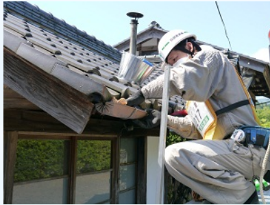
Rainwater Guttering: Removal of deposited materials
