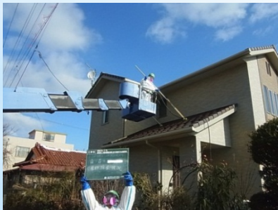
Roof: Cleaning with a brush
