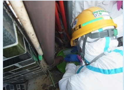
Rainwater Guttering (Downspout): High-Pressure water washing, vacuuming
