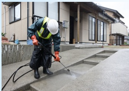
Concrete Slab: High-Pressure water washing
